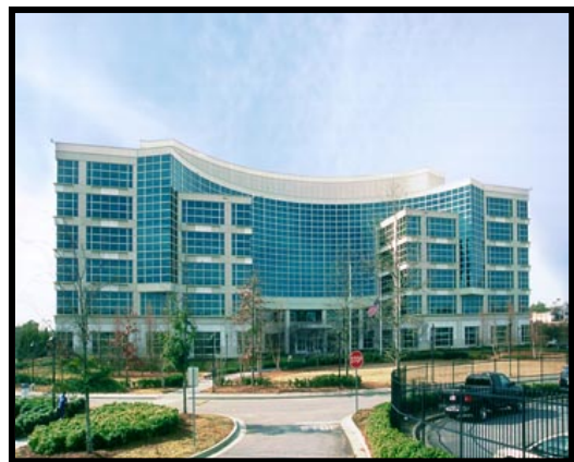
Figure 1. HGS Personnel perform Facility Maintenance at the IRS Center, Chamblee, GA.
