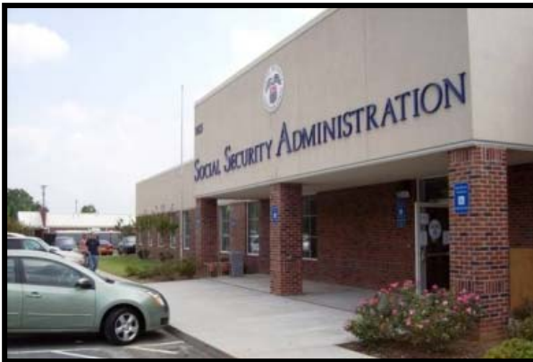
Social Security Administration Building Marietta, Georgia
